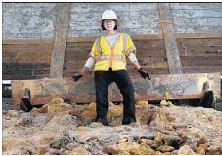
GEOLOGIST Rosalind Munro descended eight stories deep to verify the stability of the building site prior to construction.
