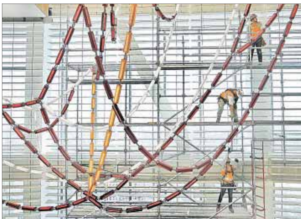
SCAFFOLDING is erected to install louvers and a three-story-high chandelier.
